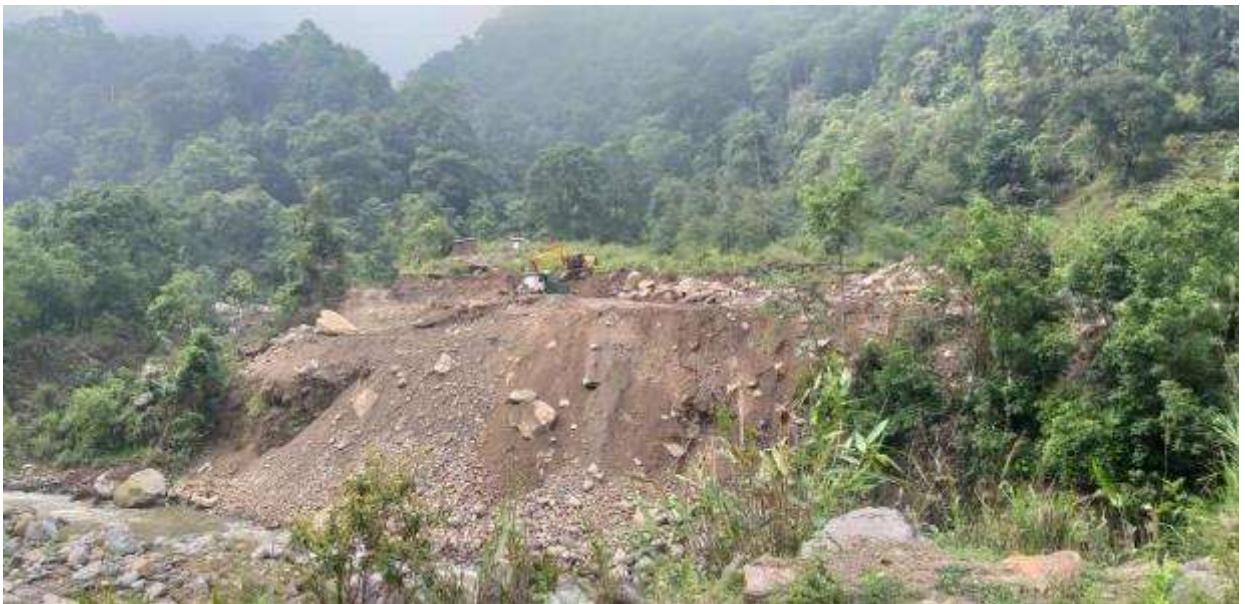
Figure 5.17: Powerhouse excavation work.
