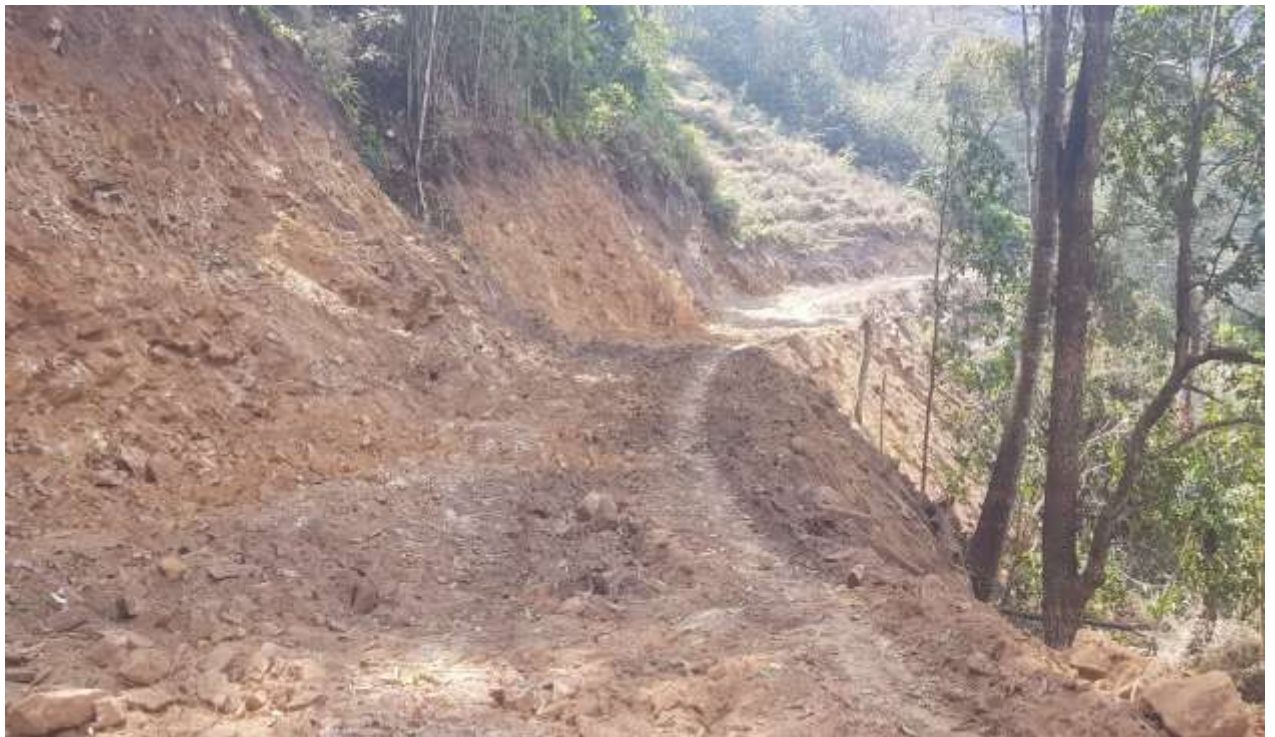
Figure 5.13:Track Widening for pipeline alignment.
