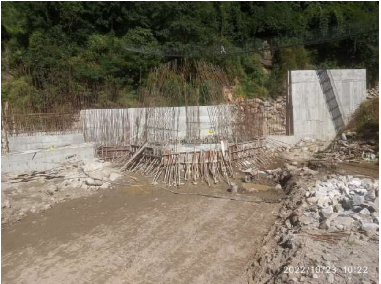
Figure 5.5: Intake, intake sluice and gravel trap area
