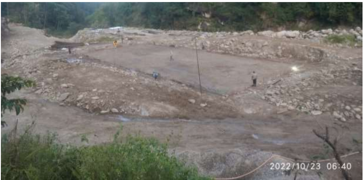
Figure 5.8: Desander area ready for PCC.
