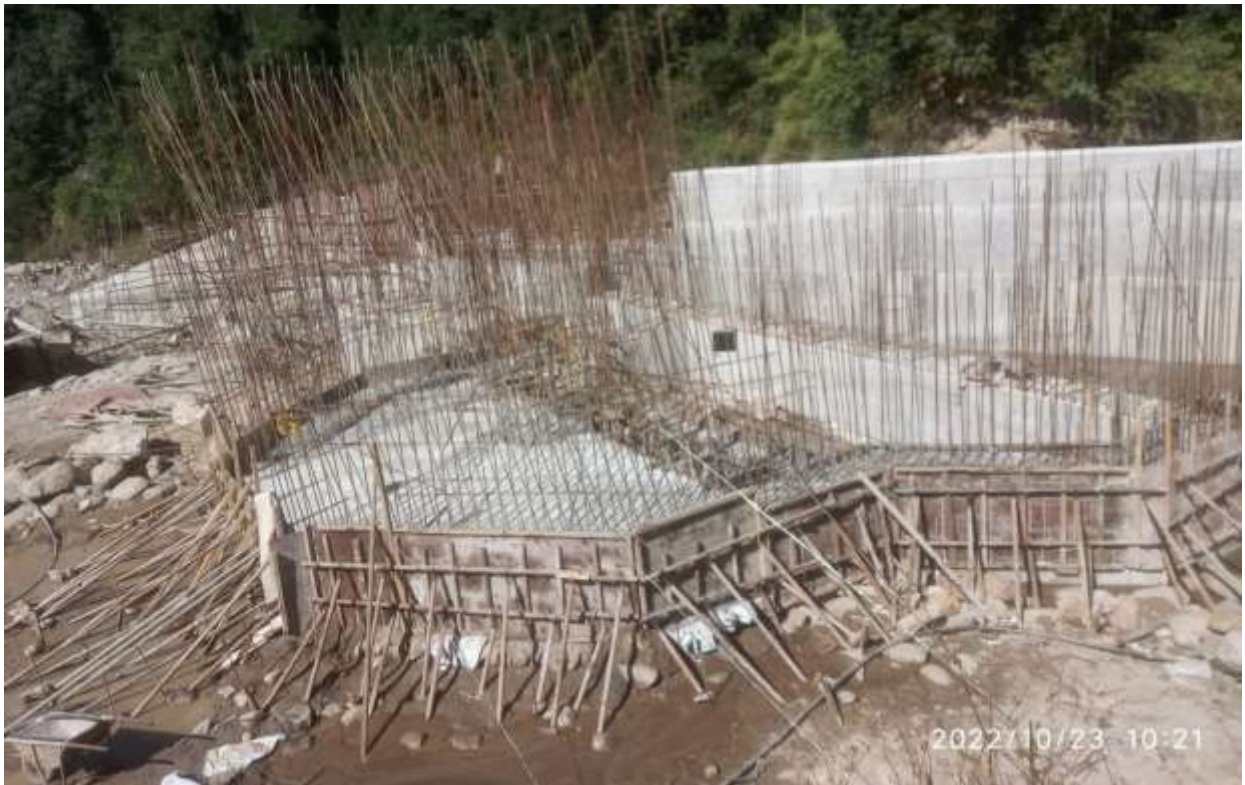
Figure 5.1: Intake slab concreting.
