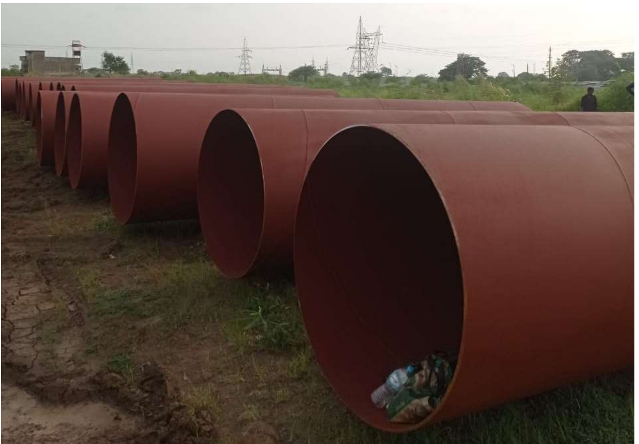
Figure 5.24: Pipes ready for transport
