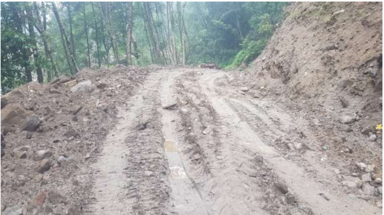
Figure 5.12:Track Widening for pipeline alignment.
