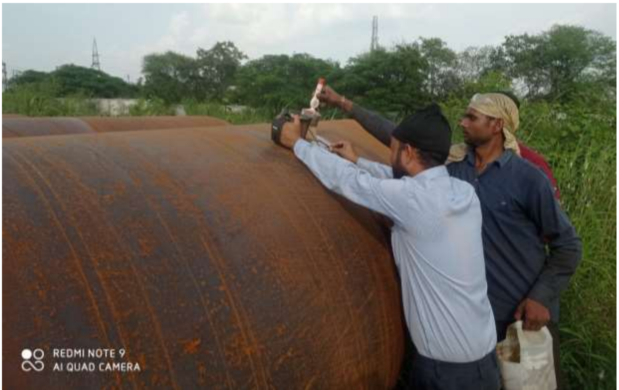
Figure 5.22: Pipe testing and supervision by client Engineer.
