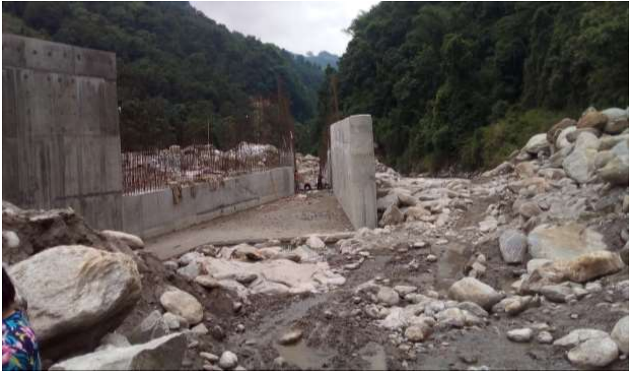
Figure 5.3: Undersluice upstream bay and divide wall.
