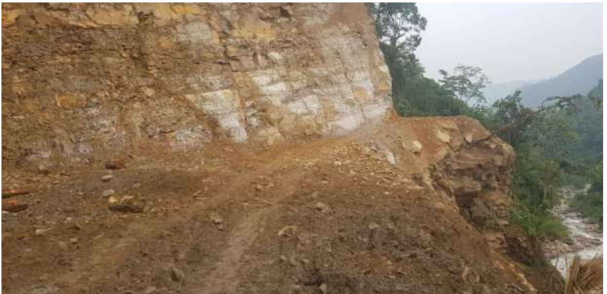
Figure 5.10: Track Widening for pipeline alignment after rocky cliff.
