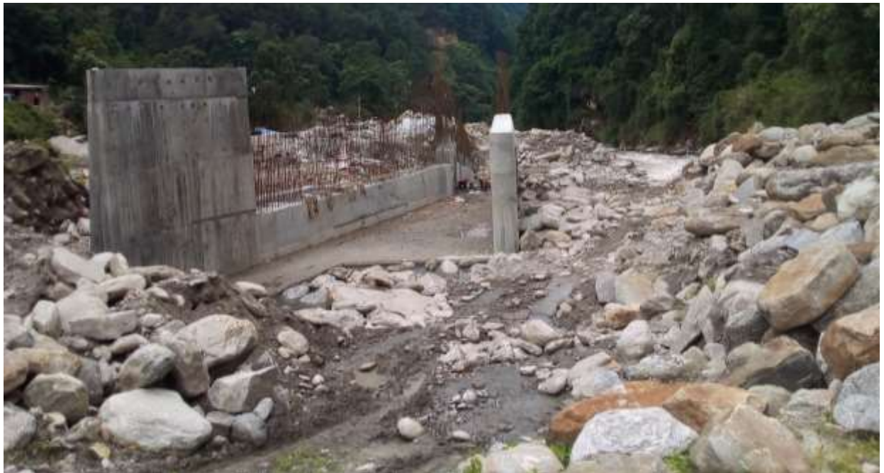
Figure 5.4: Guide wall and undersluice upstream slab from river side.
