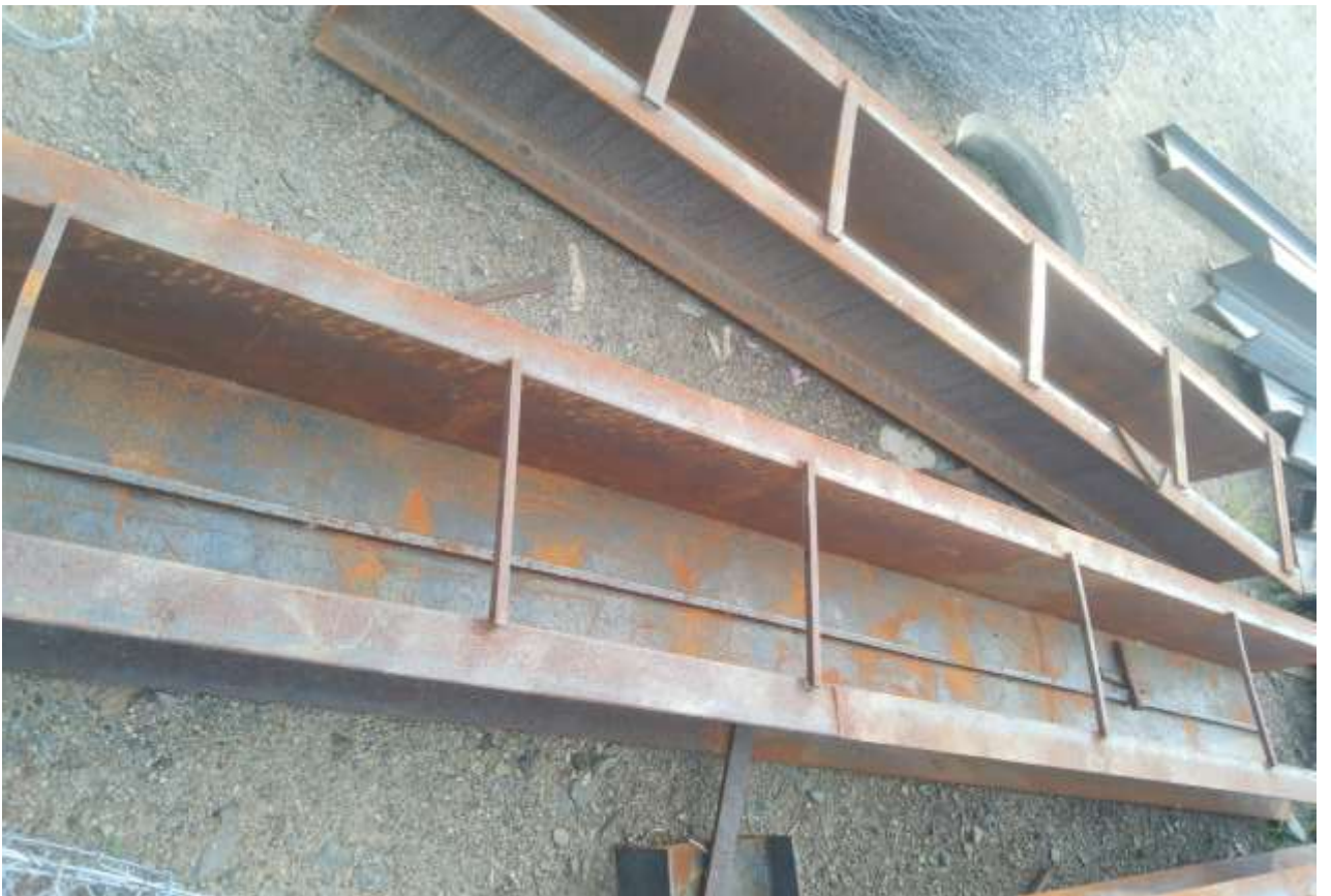
Figure 5.18: Gate frames under fabrication.
