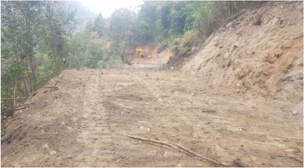
Figure 5.14: Track widening for waterway alignment.
