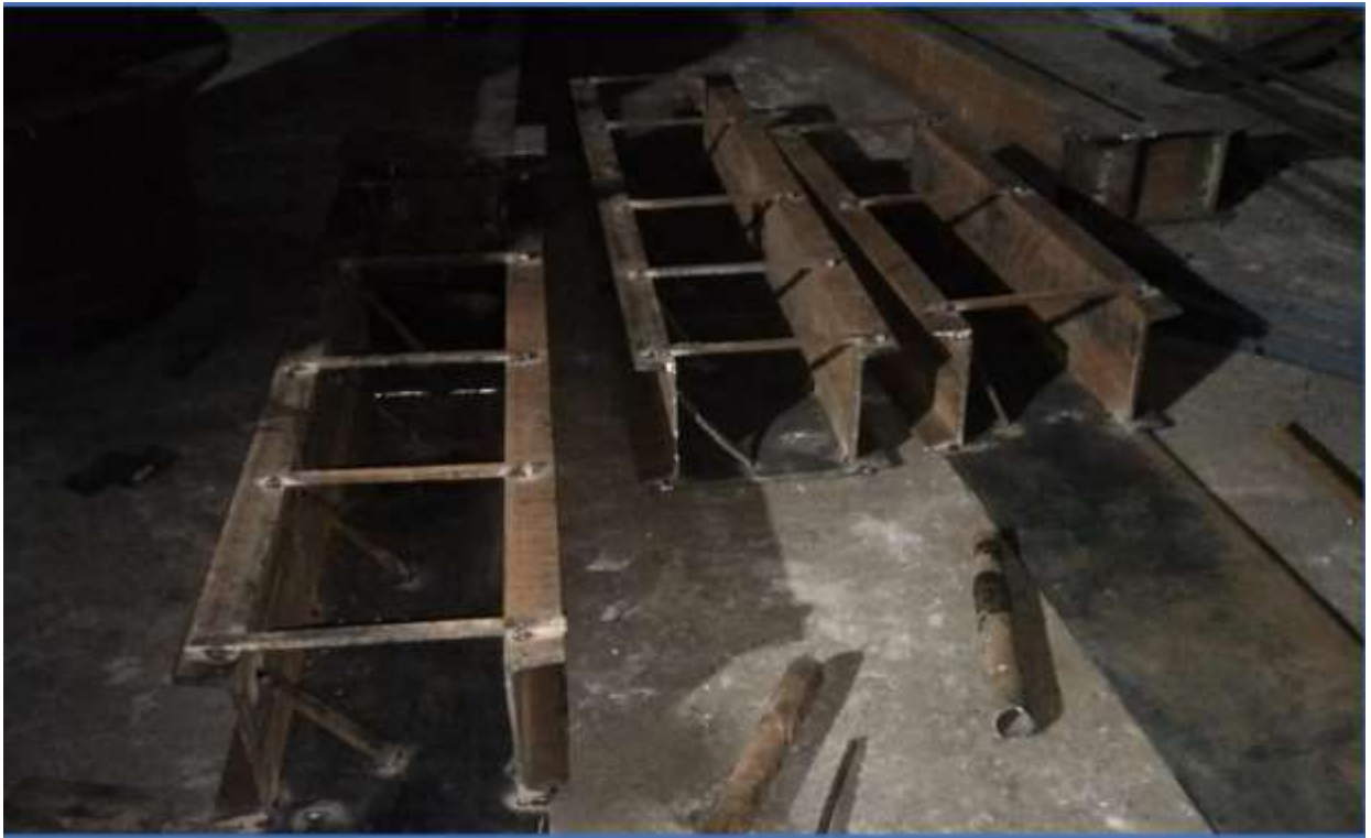
Figure 5.19: Gate Frame Under fabrication at HM contractor's workshop.
