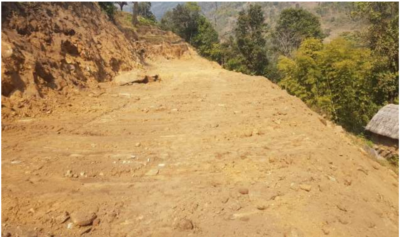
Figure 5.15: Track Widening for Headrace Pipeline Alignment
