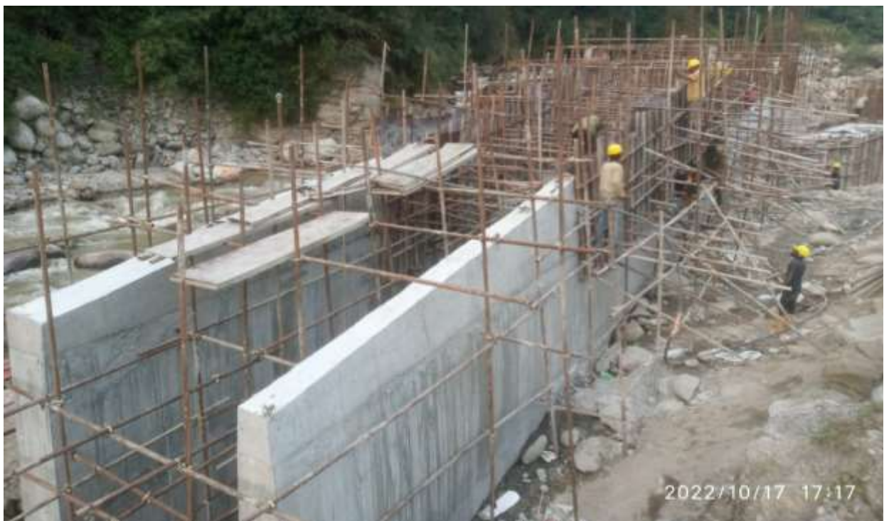
Figure 5.2: Undersluice wall from downstream
