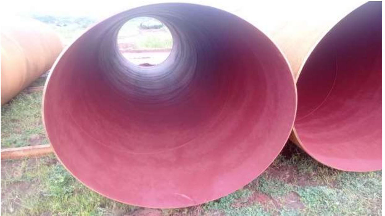
Figure 5.23: Application of zinc primer on pipe.
