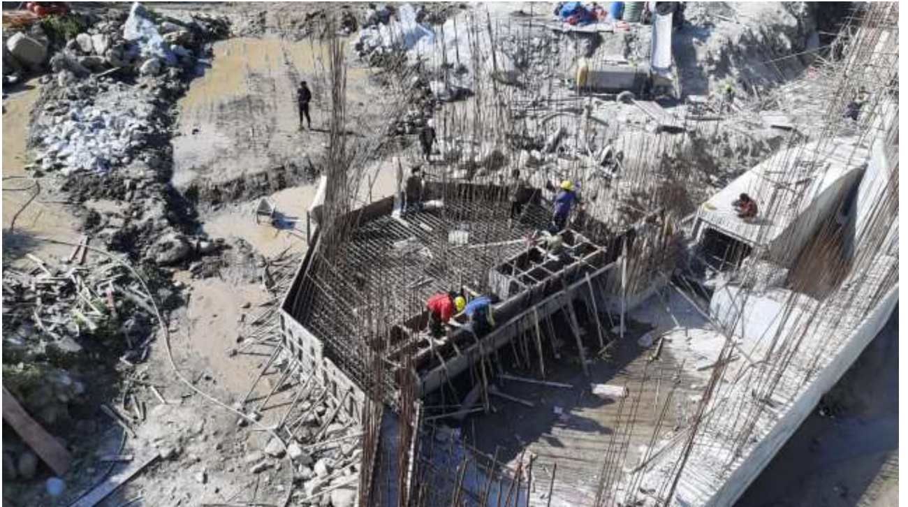
Figure 5.9: Cobble flushing channel construction.
