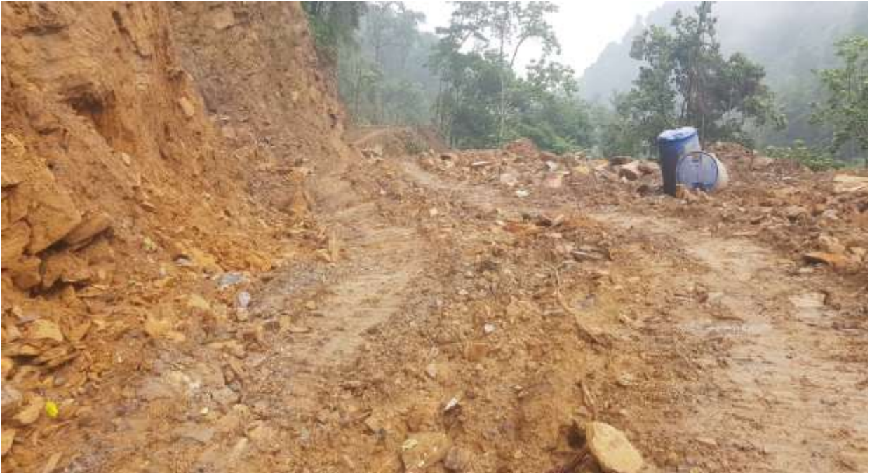
Figure 5.11:Track widening for pipeline alignment
